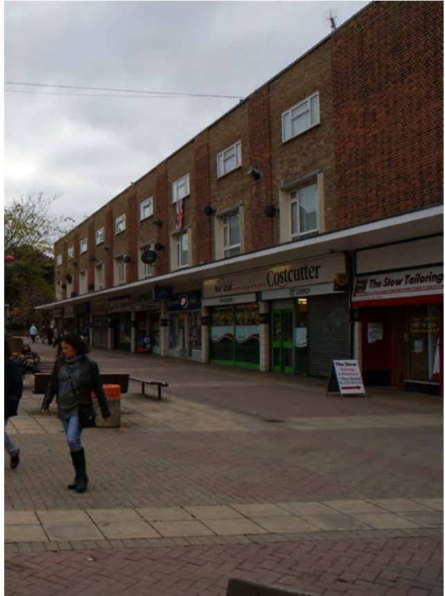
Figure 4.27: Structural canopy providing shelter and defining signage zone
