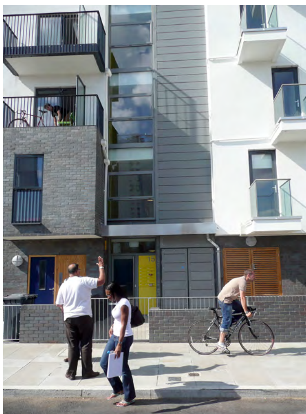
Figure 4.80: Apartment entrance articulated to add animation to the streetscape
