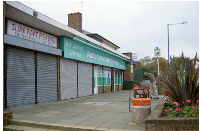
Figure 4.29: Solid external metal roller shutters can create an unwelcoming and hostile environment and should therefore be avoided
