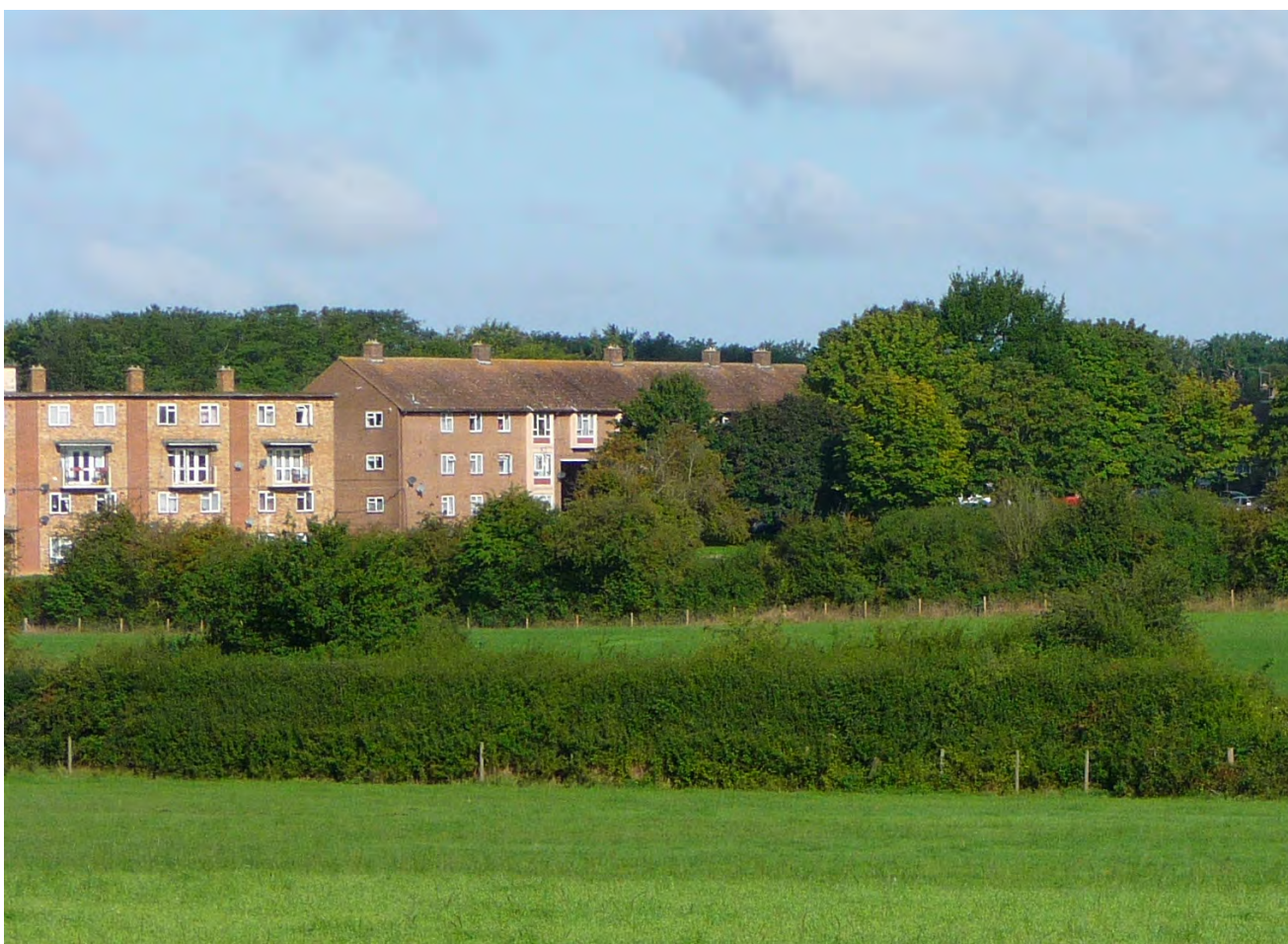
Figure 4.53: Development in Harlow providing a strong edge to a Green Wedge
