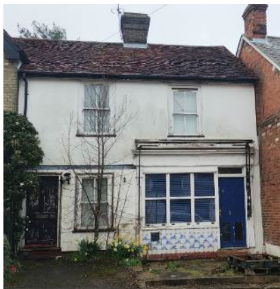
Fig. 4.5: Modification of window to become shop window
