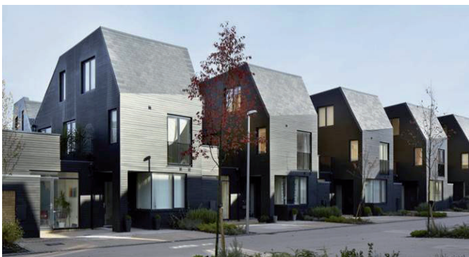
Innovative housing types at Newhall, Harlow
