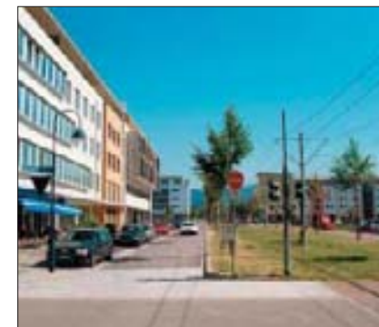
Freiburg - Development designed to maximise proximity to public transport system (grassed tracks for LRT, Freiburg)
