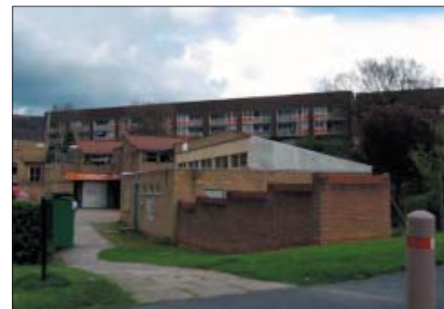
Undefined boundaries between public and private space with 'left-over' and 'un-owned' areas.
