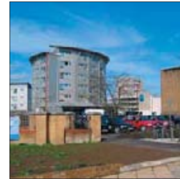
Confused pattern of buildings and uses within the Town Centre (Harlow)
