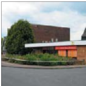
Poor performing local 'Hatch' (Harlow)
