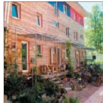
Cycle provision integral to residential development (Freiburg)
