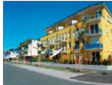
Freiburg - Residential development providing a clear articulation of street edge
