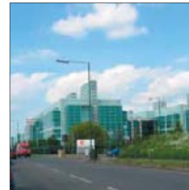
Large scale modern office space affects the overall character of local places. Tendency for human scale in design to be overlooked (Pinnacles, Harlow)
