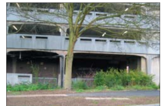
Inactive and poor quality buildings in the Town Centre
