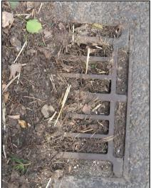
**Improve maintenance of the drainage network:** Drainage maintenance schedules should be evaluated to reflect the findings of this study. The potential for blockages in the drainage network would exacerbate surface water flooding; this would be a particular issue in all the areas predicted to be at risk of surface water flooding during an extreme event. It is recommended that a risk-based approach is applied so that drainage infrastructure in key areas is kept clear and maintained.
