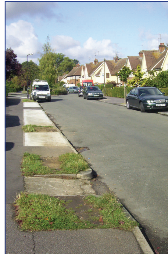
Unsympathetic street materials used for on-street parking along Manor Road which have a detrimental impact on the character of the conservation area.
