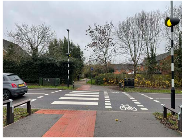
Figure 73 Parallel zebra crossing at Church Langley Way
