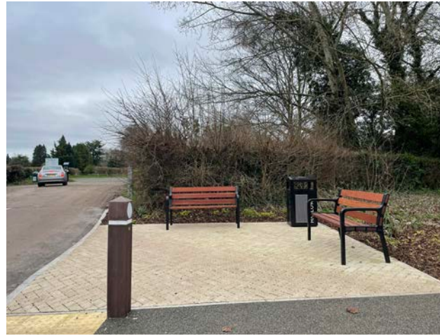
Figure 9 New seating area provided as part of the North-to-Centre STC scheme
