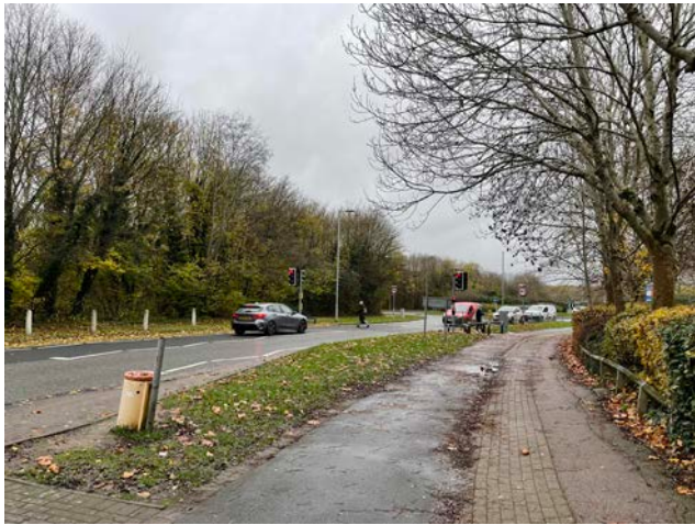
Figure 71 Signalised crossing outside Tesco
