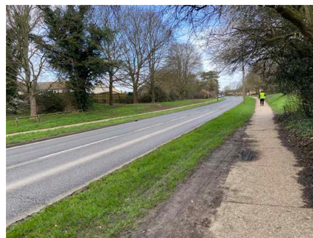
Figure 44 Lack of cycle provision along Howard Way
