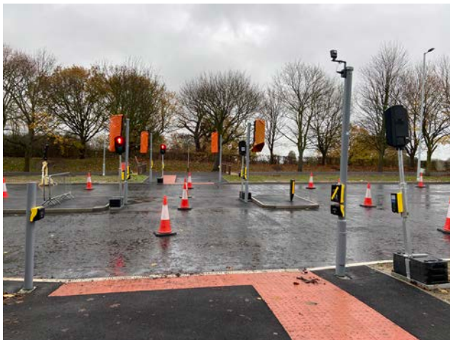
Figure 62 New toucan crossing along the north-to-centre STC
