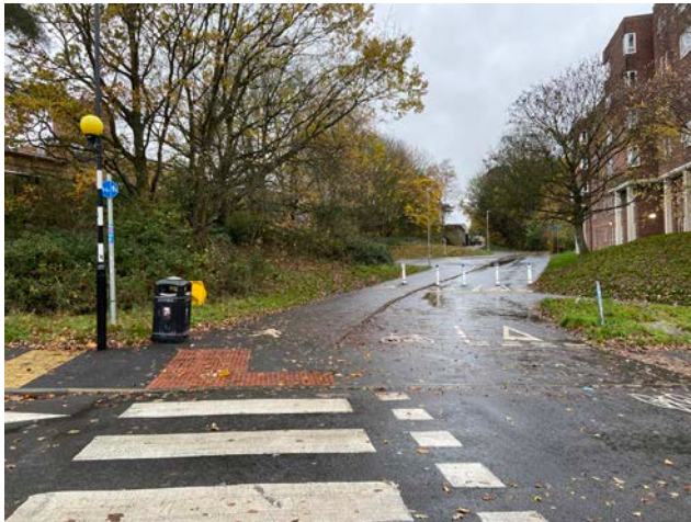
Figure 52 Parallel crossing, Hodings Road (Harlow)
