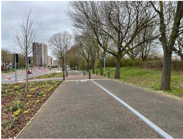
Figure 7 New footpath and cycleway as part of the North-to-Centre STC scheme
