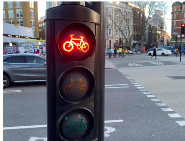
Figure 53 Dedicated cycle signal at junction (Old Street, London)
