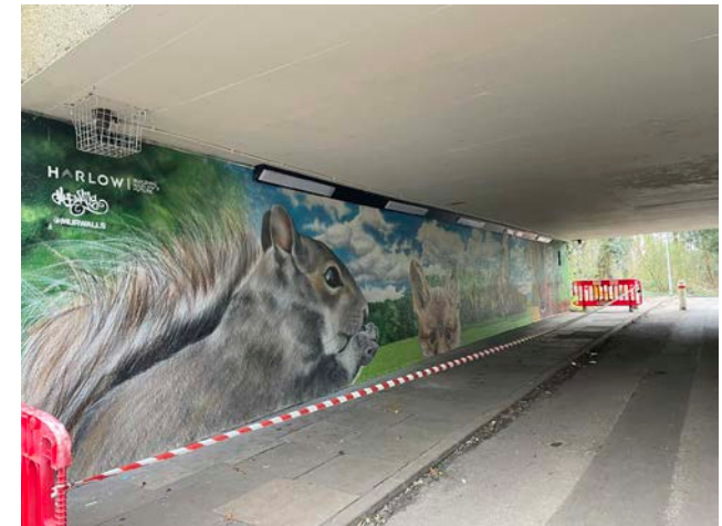
Figure 57 Upgrades to existing underpass (Nettleswell Road, Harlow)
