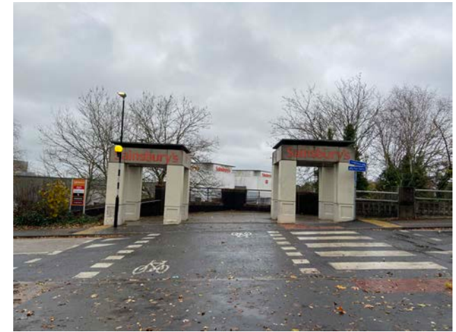
Figure 61 New parallel zebra crossing connecting Sainsbury's on Hodings Road
