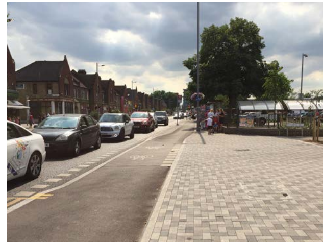
Figure 49 Continuous footway and cycle track, Hitcham Road, Waltham Forest
