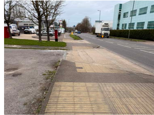
Figure 37 Lack of priority at side-road junctions along Elizabeth Way cycle track
