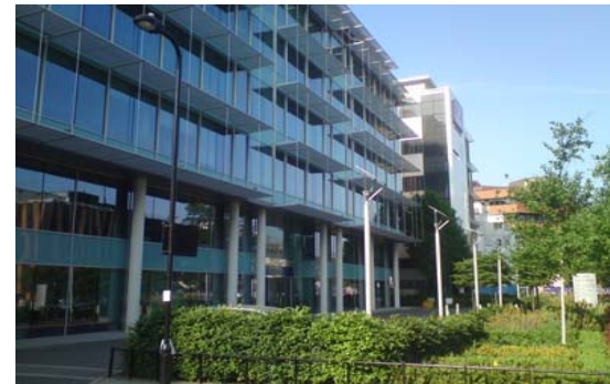
Photo A - Hedge screening of frontage parking
