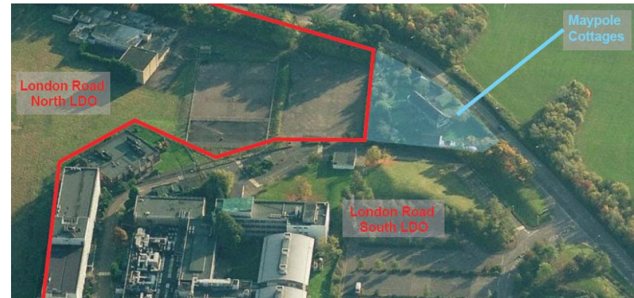
Photos showing proximity of Maypole Cottages to the LDO boundary.
