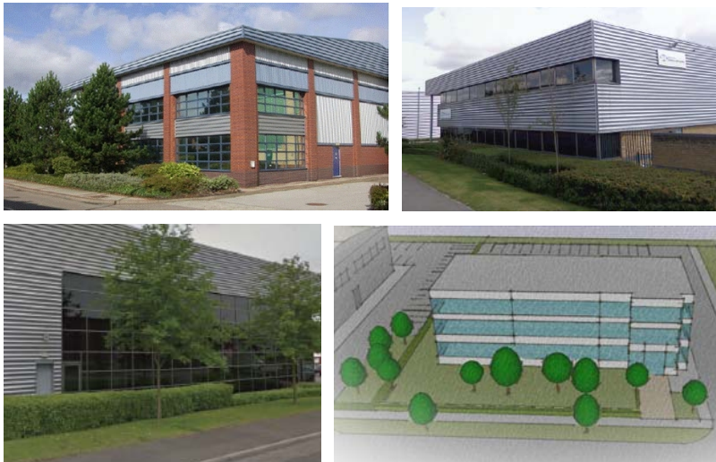
Front boundary landscaping helps to provide an attractive business park environment
