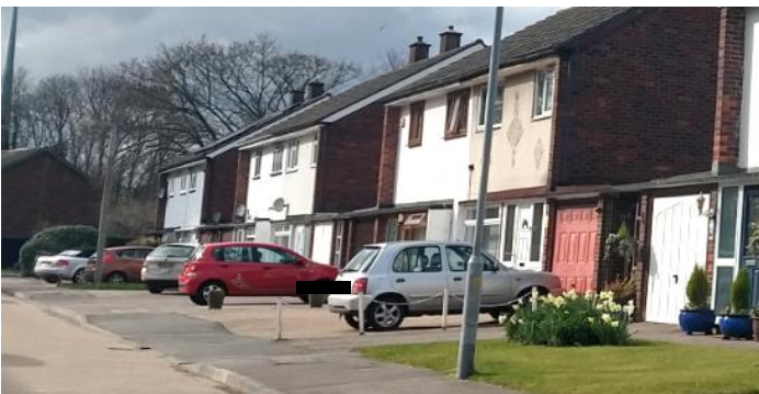
Fig. 8.c.6: Gardens converted to hardstanding
