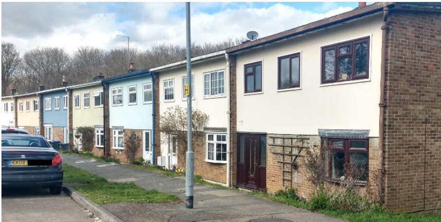
Fig. 15.19: Gardens converted to hardstanding and door/window frames in darker colour, Tany's Dell
