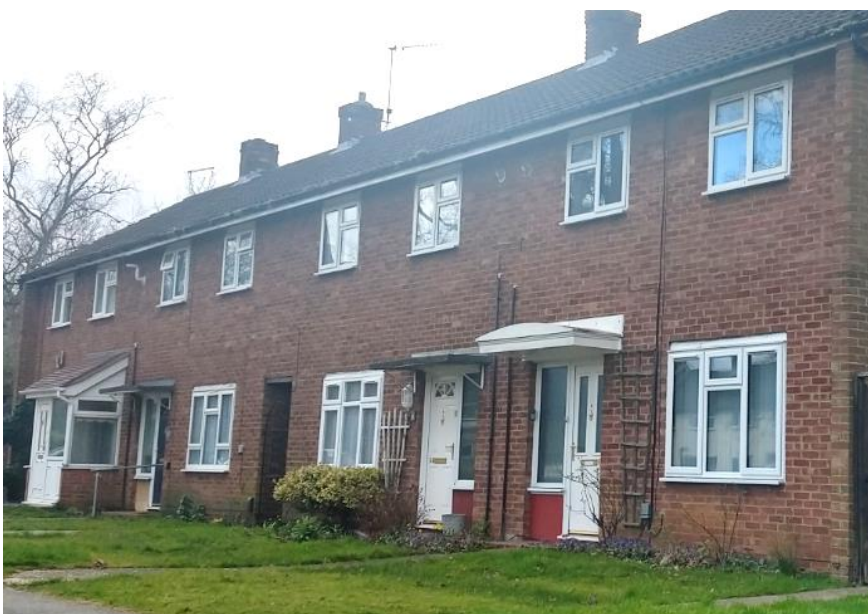
Fig. 15.14: Canopy extension and porch construction, Great Plumtree
