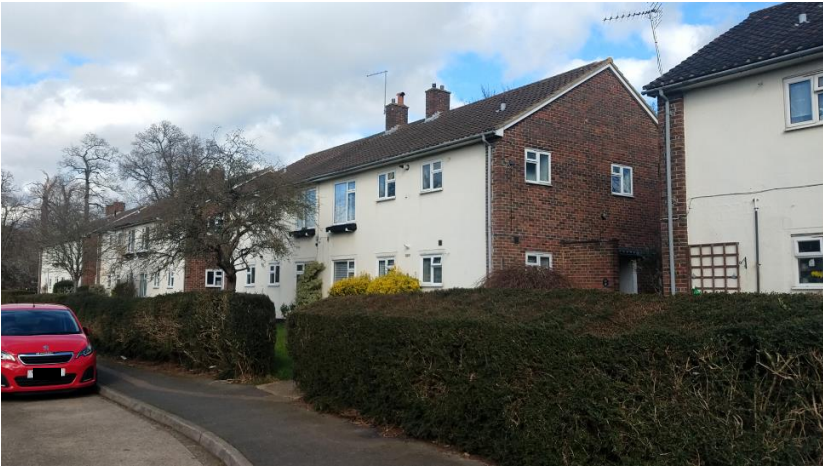
Fig. 4.o.1: Blocks of flats
