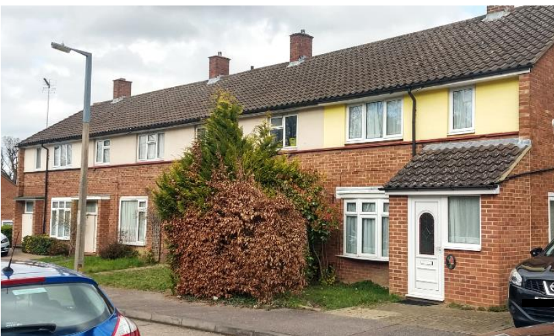
Fig. 15.8: Facade in contrasting colour, Fesants Croft
