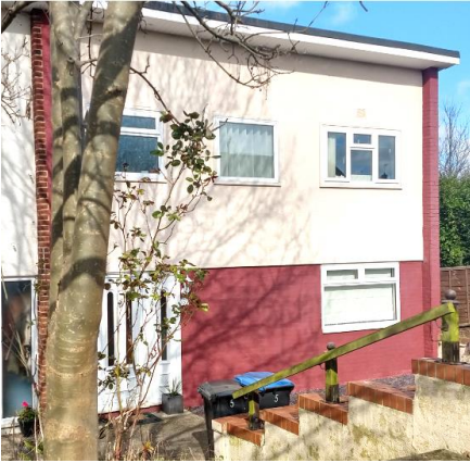
Fig. 7.b.2: Exposed brick painted
