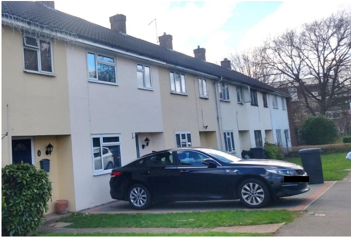
Fig. 8.a.7: Garden converted to hardstanding
