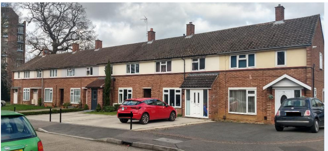
Fig. 15.11: Porch constructions and gardens converted to hardstanding, Fesants Croft
