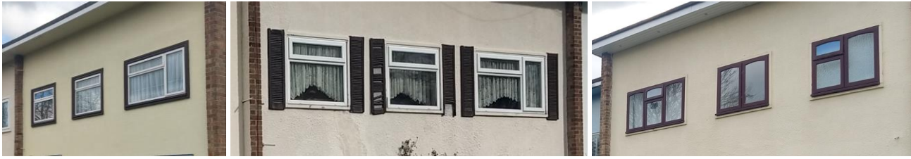
Fig. 12.a.3: Brown-framed windows; additional features
