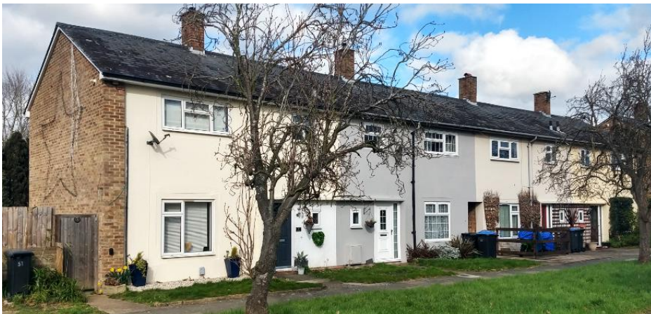
Fig. 15.4: Facades in contrasting colours and doors/window frames in a darker colour, Broomfield
