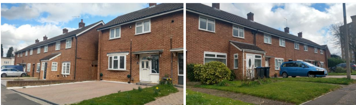
Fig. 8.b.5: Gardens converted to hardstanding
