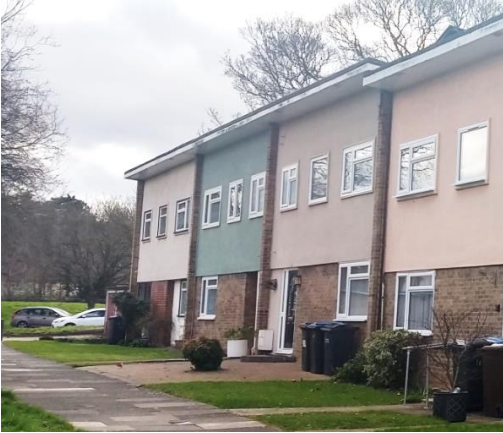
Fig. 12.a.11: Garden converted to hardstanding
