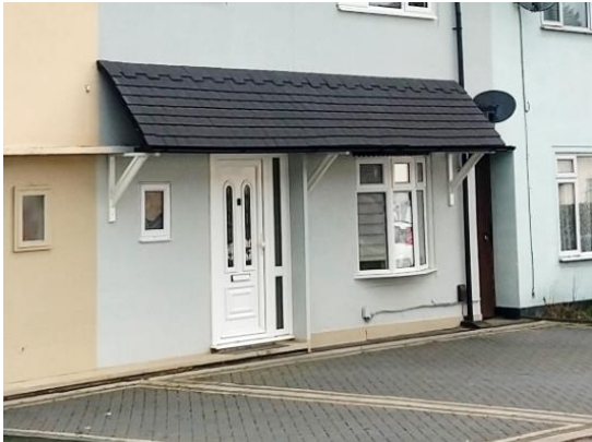
Fig. 9.b.3: Large canopy construction
