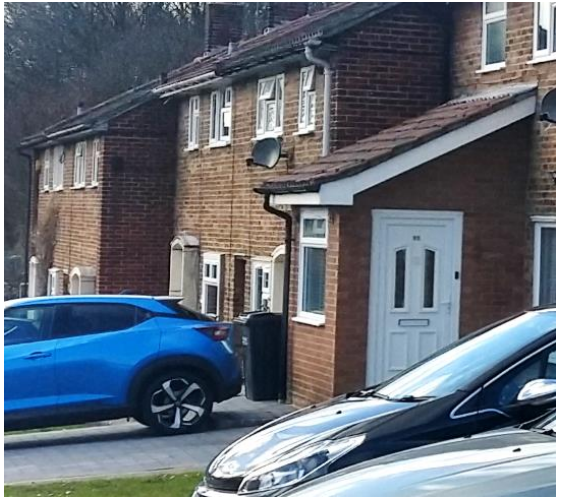
Fig. 4.b.3: Canopy converted to porch
