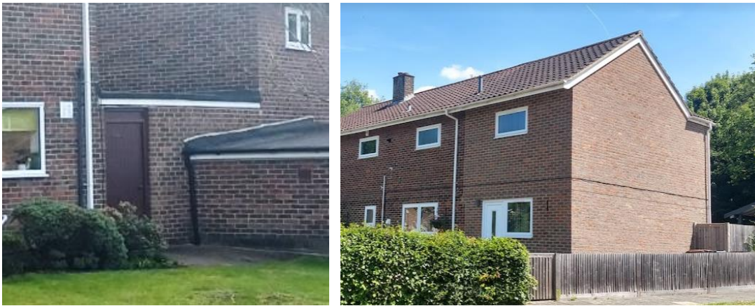
Fig. 4.c.4: Annex linking houses Fig. 4.c.5: Annex first-floor extension
