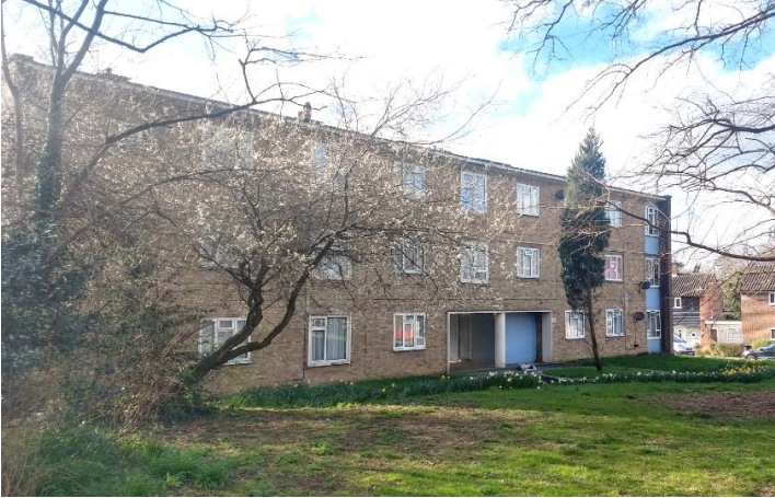
Fig. 9.o.2: Three-storey flat block – rear elevation
