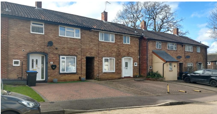
Fig. 9.c.4: Gardens converted to hardstanding
