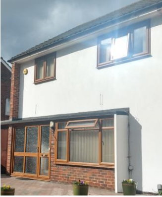
Fig. 8.c.2: Brown-framed windows and door
