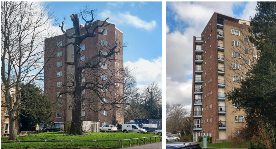
Fig. 14.1: The Lawn tower block
