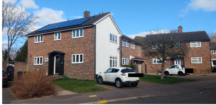
Fig. 9.a.6: Front gardens partially converted to hardstanding
