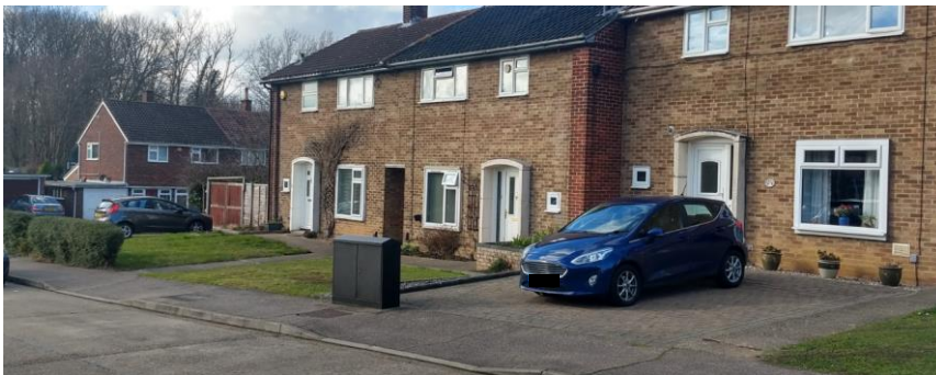
Fig. 4.b.3: Gardens converted to hardstanding
