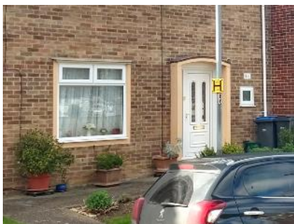
Fig. 9.c.2: Repainted canopy and window frame
