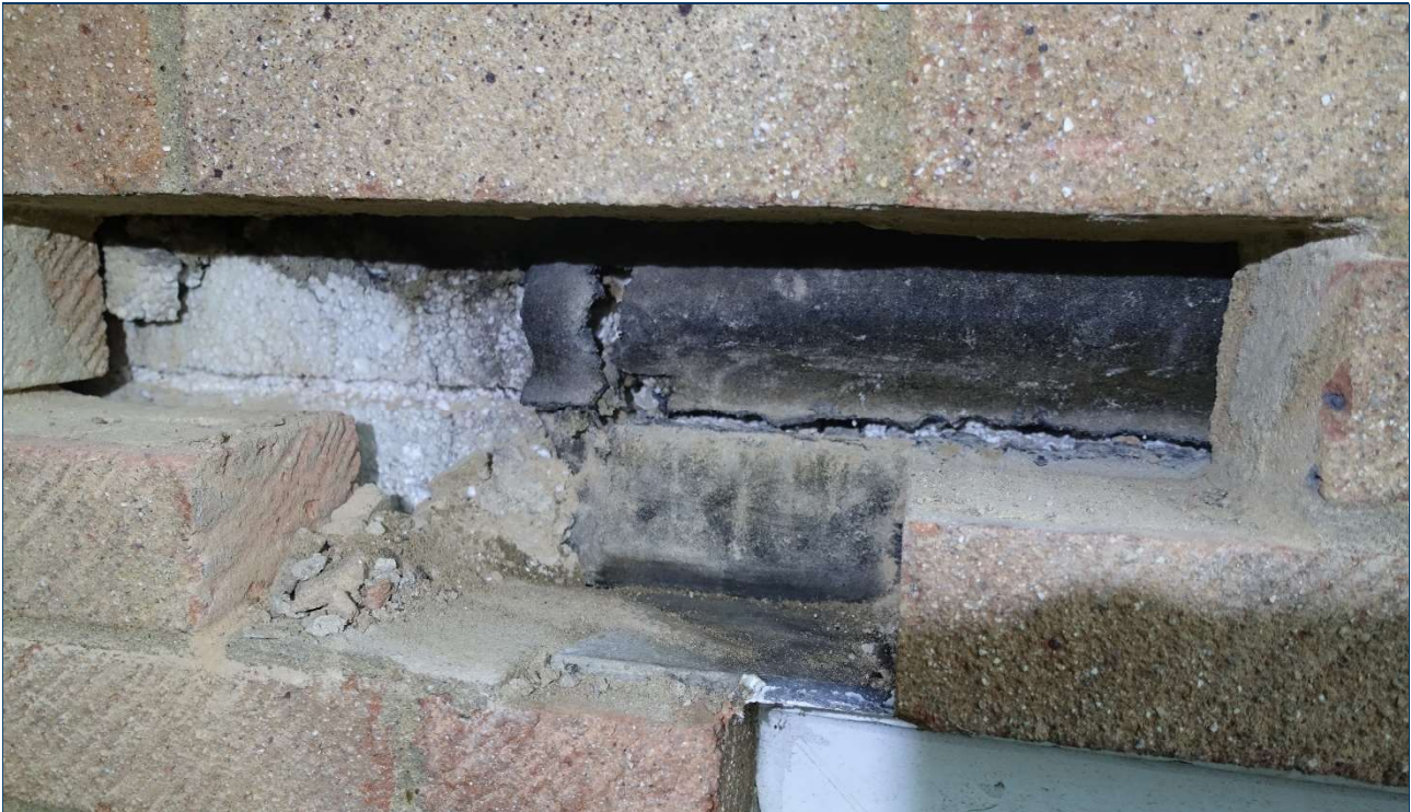
Photo 17 Window Head Detail – Bitumen Type DPC Cavity Tray without Stop End
