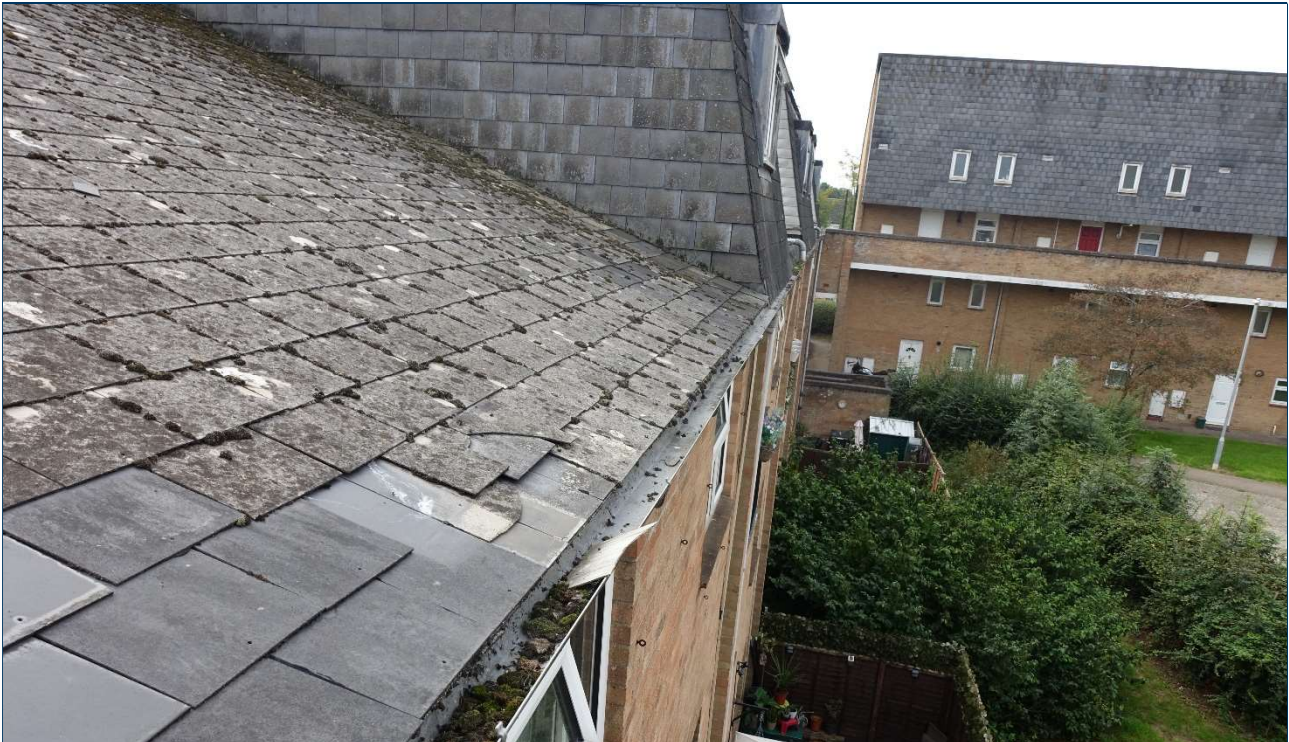
Photo 05 Mono-Pitch Roof – Debris / Tile in Gutter
