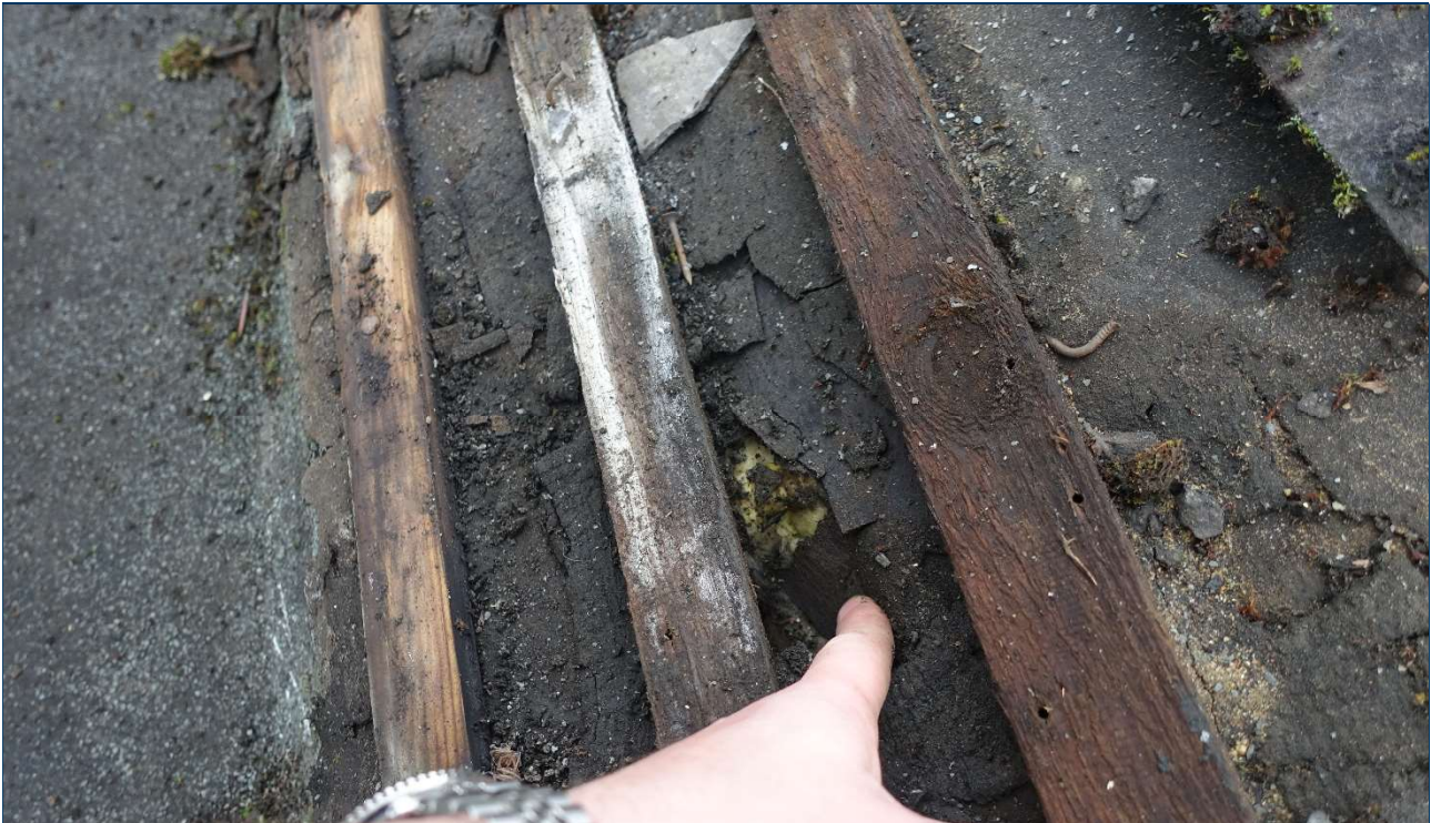
Photo 09 Mono-Pitch Roof – Damage to Underlay & Saturated / Decayed Battens
