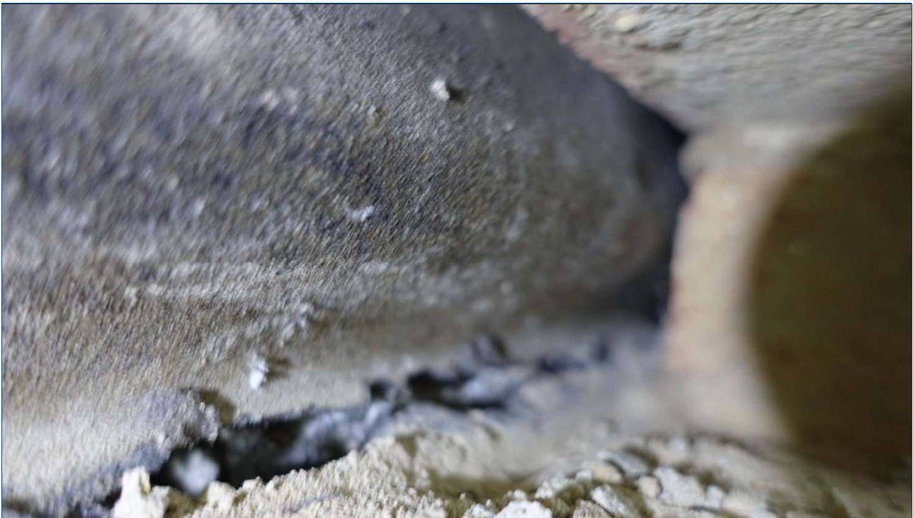
Photo 18 Window Head Detail – Bitumen Type DPC Cavity Tray
