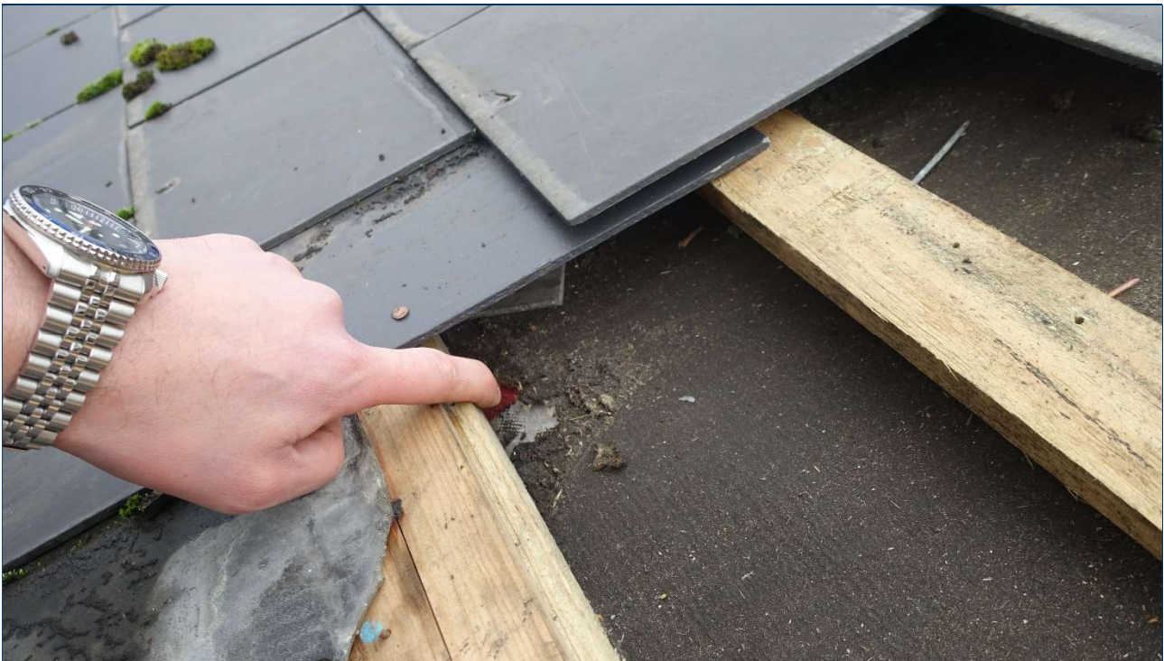
Photo 08 Mono-Pitch Roof – Damage to Underlay
