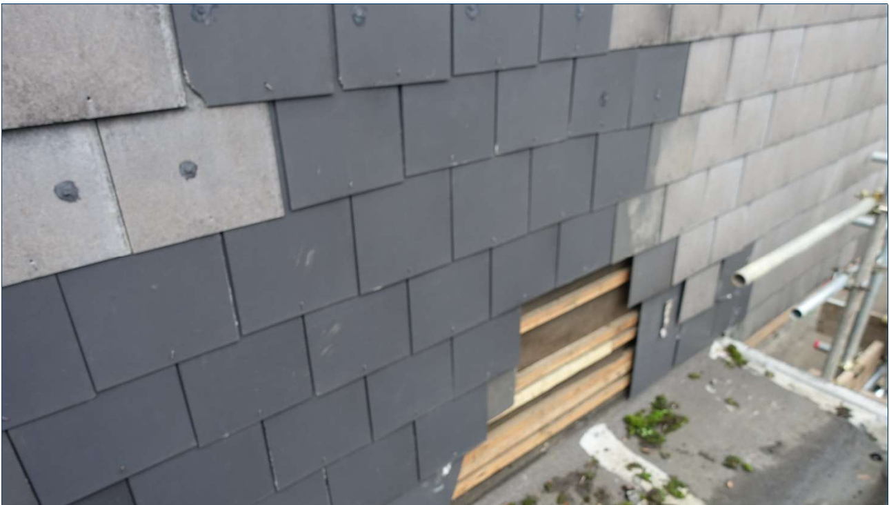
Photo 12 Vertical Wall Cladding – Area No.1 Exposed
