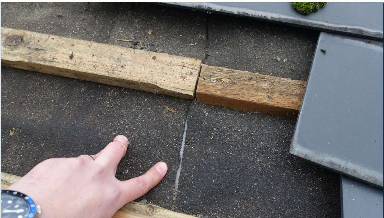
Photo 10 Mono-Pitch Roof – Underlay Butt Joint
