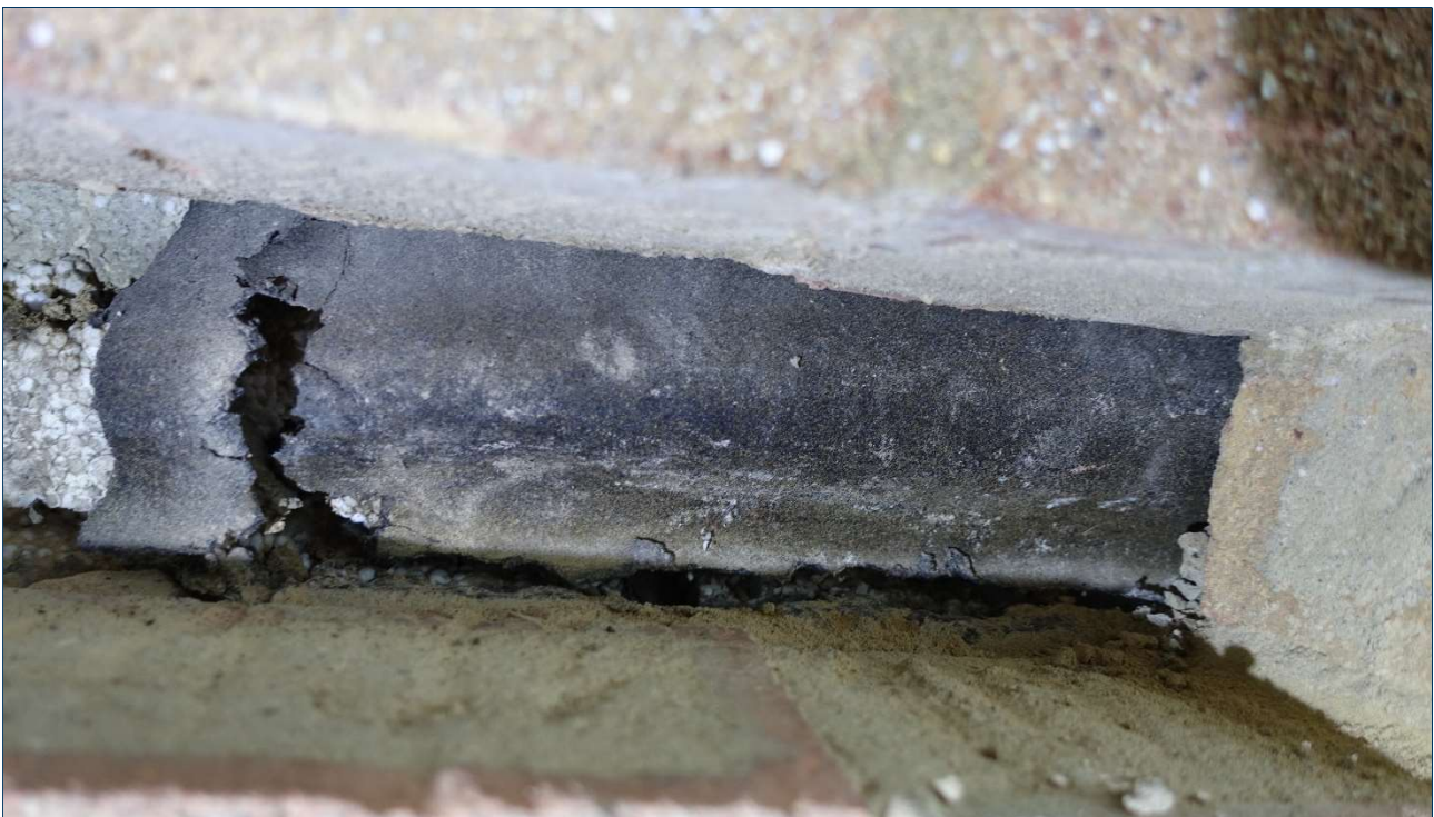
Photo 16 Window Head Detail – Bitumen Type DPC Cavity Tray
