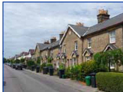
Consistent building lines along Bury Road
