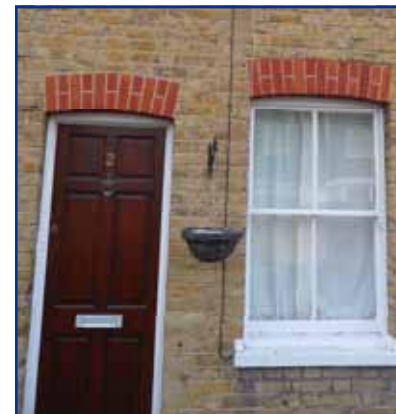
Gauged brick lintels on Mulberry Terrace
