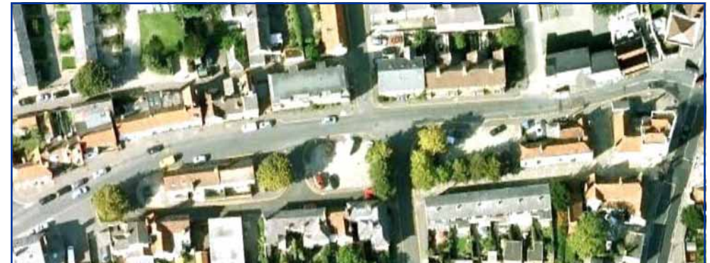
Market Street & Fore Street, 2011 - showing demolition of infill development between Market St and Fore St (Source; Google Earth)
