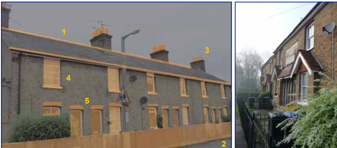
Mulberry Terrace (left) - features which provide a horizontal and vertical emphasis are highlighted in orange which provide a pleasing composition. Bargeboards on Oddfellows Terrace (right)
