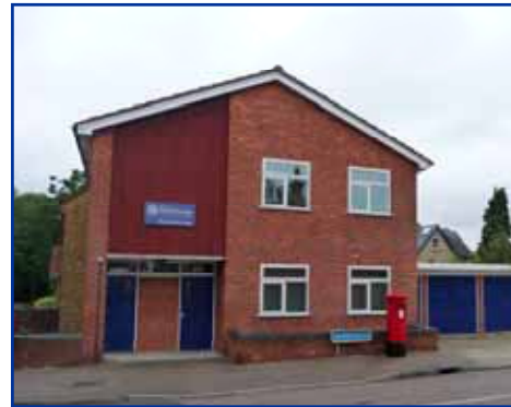
Building at the termination of the view along Market Street looking west
