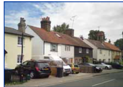
Eroded front garden boundaries on the eastern side of the High Street
