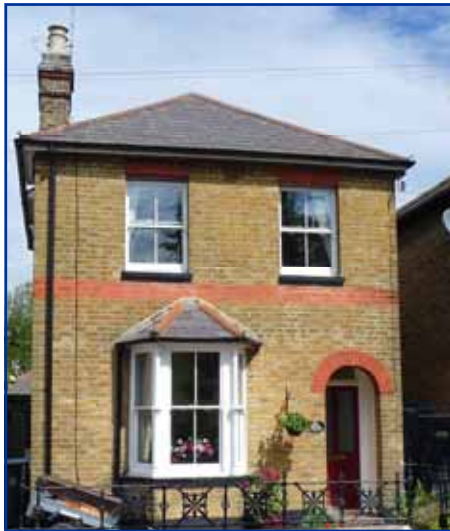
Decorative plastering above doors and windows
