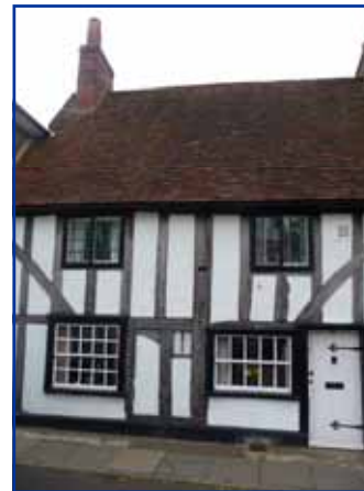
Timber Frames, 17 Fore Street
