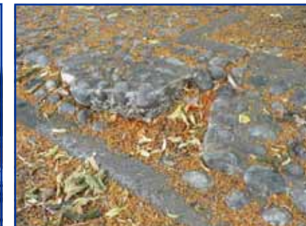
Maintenance of pavements, Fore Street
