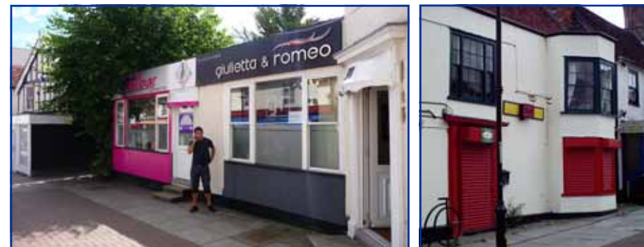
Above a range of unsympathetically designed shop fronts along Old Harlow High Street in terms of materials, colours and security shutters
