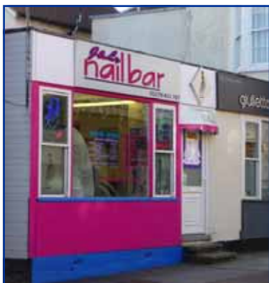
Unsympathetically designed shop fronts in terms of style, materials and colour
