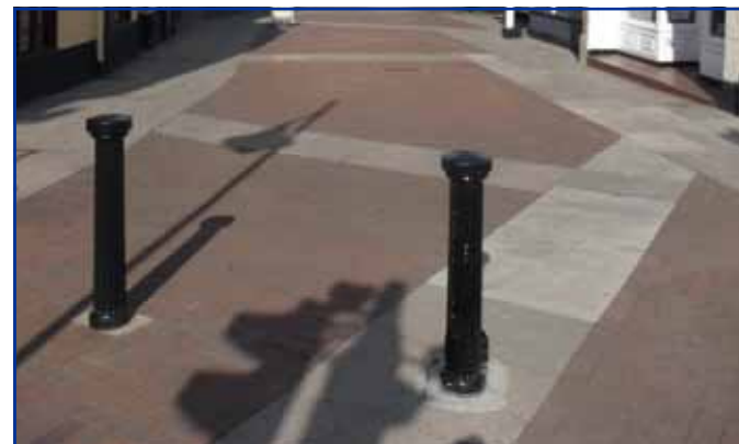
High Street - Cast iron bollards finished in black
