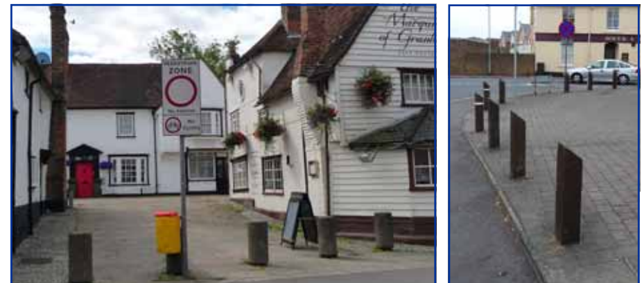
Fore Street / Market Street
