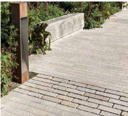
Figure 56 Permeable paving can be positive where subsurface conditions restrict planting
