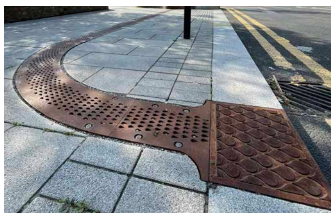
Figure 128 Drainage inlet cover highlights its purpose for SuDS stormwater capture. Haringey rain gardens by Robert Bray Associates
