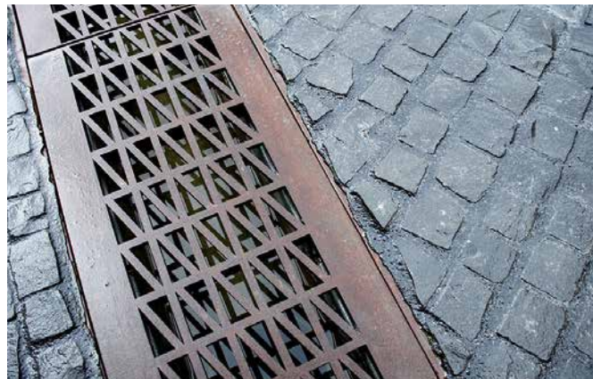
Figure 126 Drain detail in BRFkredit plaza, Copenhagen © landskab.dk
