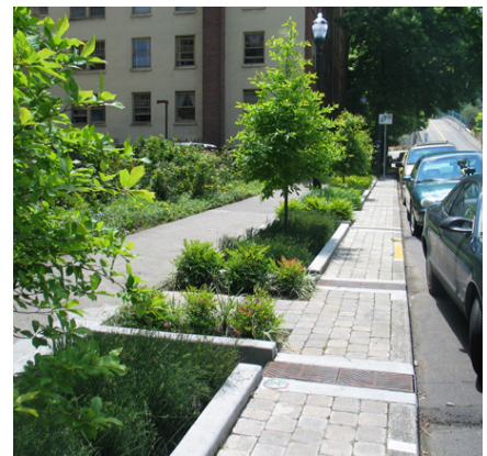
Figure 60 Rain gardens with water inlets capture surface water runoff from the adjacent carriageway. 12th Street Avenue by City of Portland
